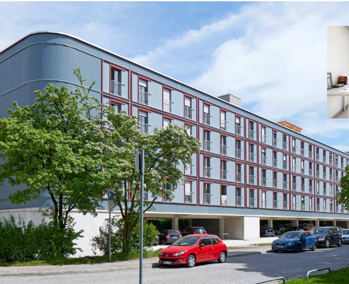
LIVING NEXT TO DANTEBAD The four-story building rests on stilts above an existing car park. This means no natural ground had to be sealed.
